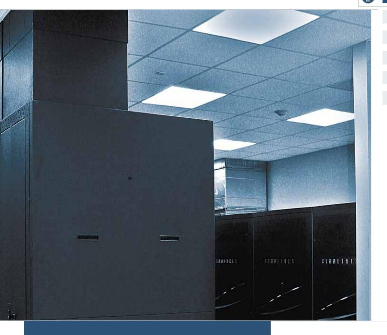
Attaching the racks firmly together provides strength, stability, and allows cabling to pass between racks. Side panel sets are available to cover the sides once the installation is complete; one set of side panels will close off an entire row of ganged racks.
